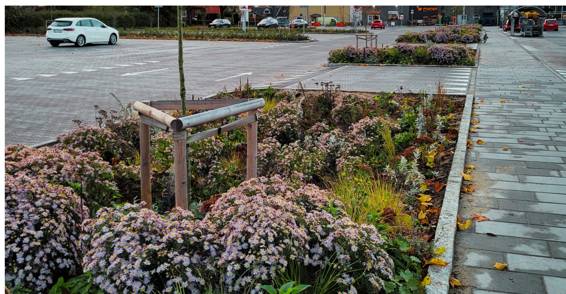
Raingarden with filter soils integrated into the roads and car parks
