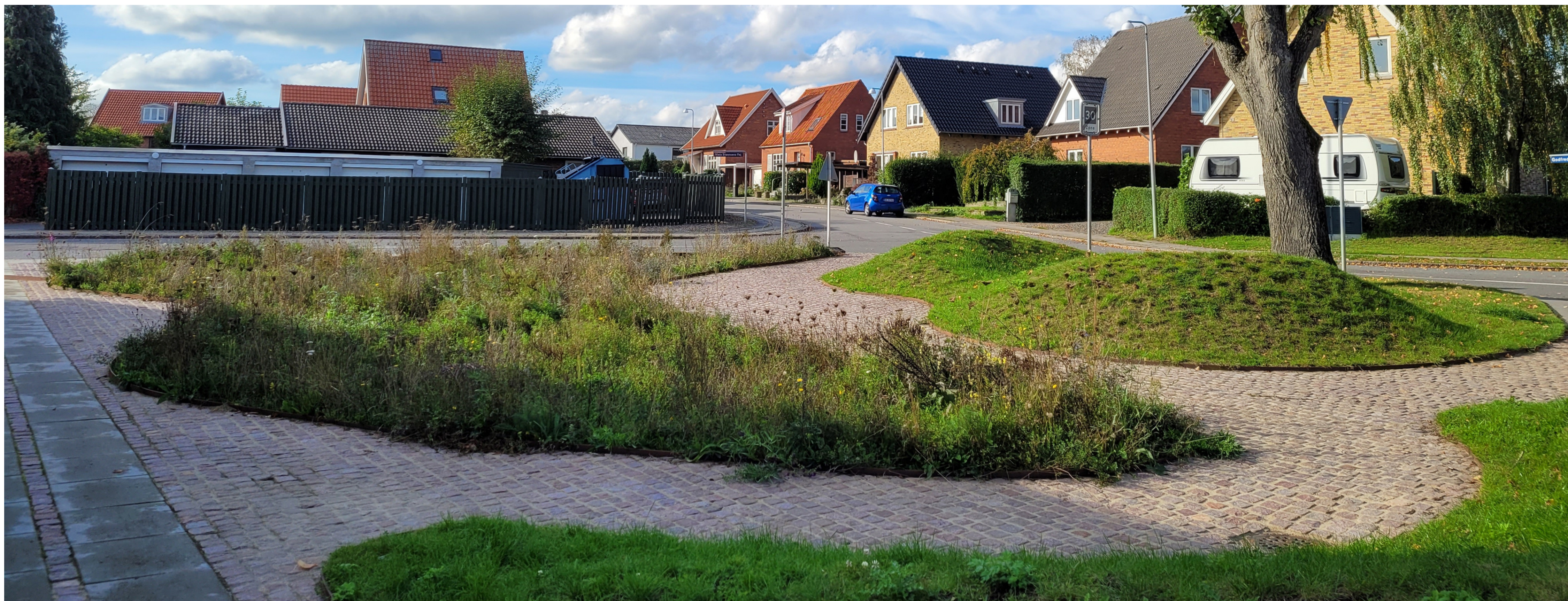
Filter vegetation and soil implemented at newly constructed housing areas in Bolbro
